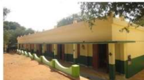
Classrooms constructed under the GGP grant
