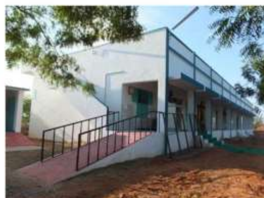
The center constructed under the GGP grant
