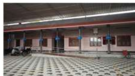
A hostel constructed under the GGP grant
