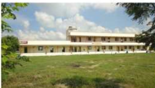
A school building constructed under the GGP grant
